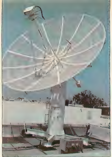
On the roof: Dish antenna downlinks satellite photographs.
